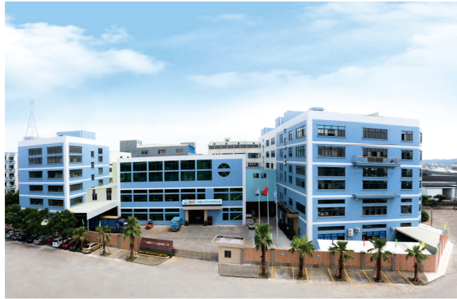
碧麗公司總部基地 The headquarters base of Bili Company
